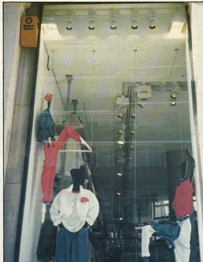
Vertical and horizontal lighting track is used to light a window by Esprit, London. It carries Eclipse low voltage spotlights by Erco.
