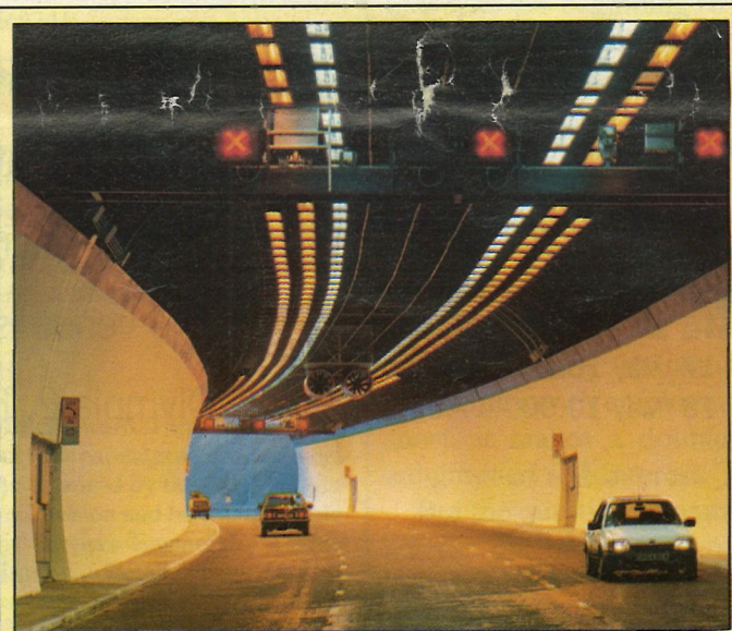
Some 1200 special extruded aluminium lanterns light the tunnel linking Devon and Cornwall on the A38 bypass at Saltash.
